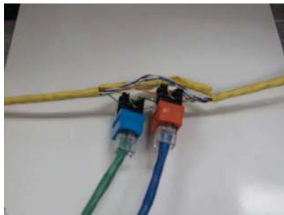
Figure 10. Wiretap covertly using single pair insulation-displacement connectors
