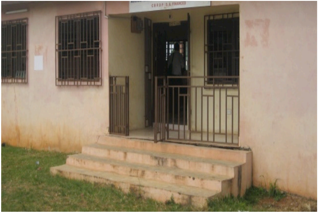
Photo 7.1: Exterior of the Aboloo CBRDP library.
