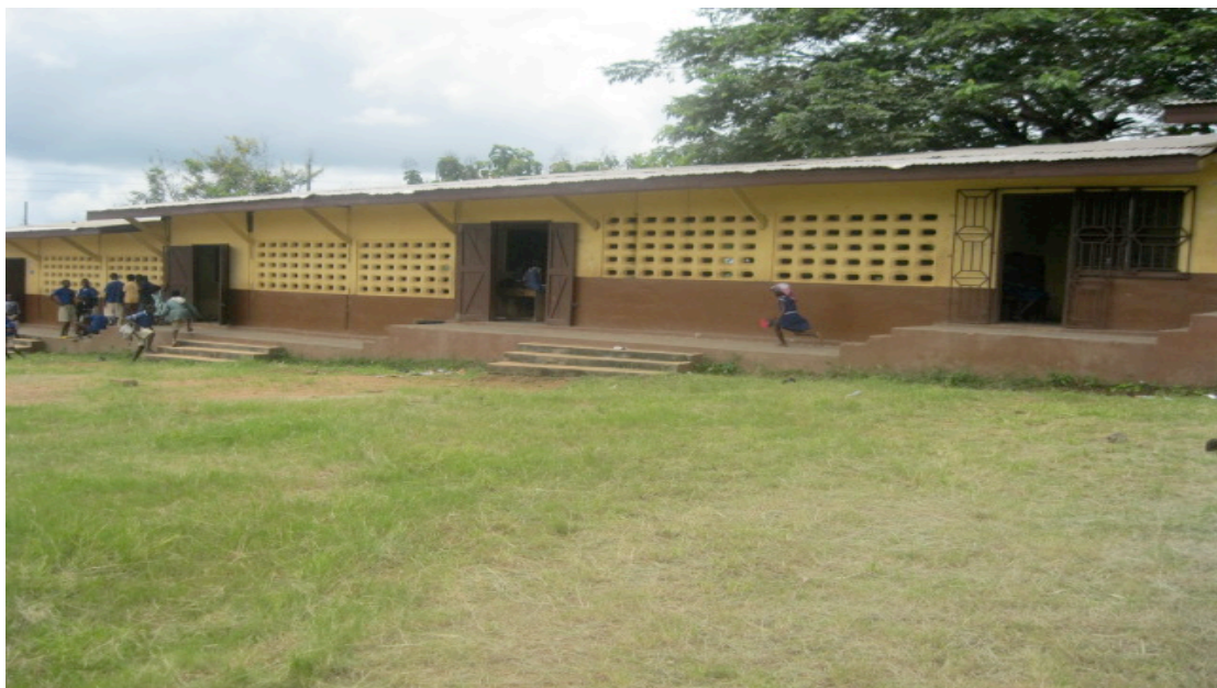
Photo 6.3: The renovated Tashie Presby School
