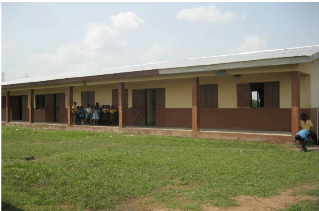
Photo 6.6: The Agbetor CBRDP Three-Unit Classroom Block.
