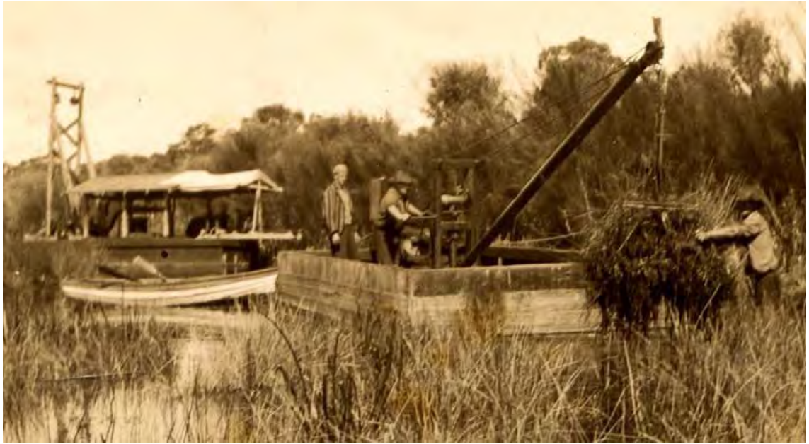
Figure 35: Dredging Loch McNess. c.1930s.
