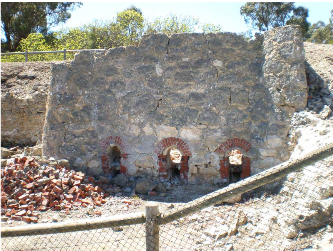
Figure 30: Limestone Kilns – Wanneroo Road, Neerabup. Source: Author, September 2012.
