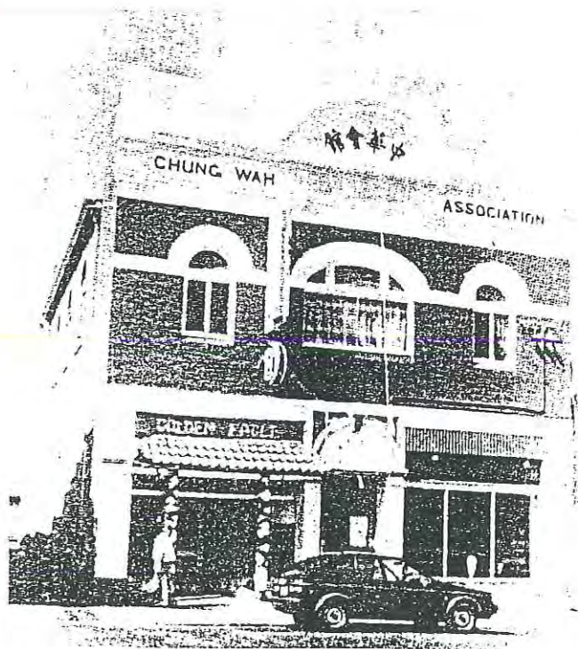
Figure 6.3 Two Pictures of the Chung Wah Hall Building Source: The Chung Wah Association
