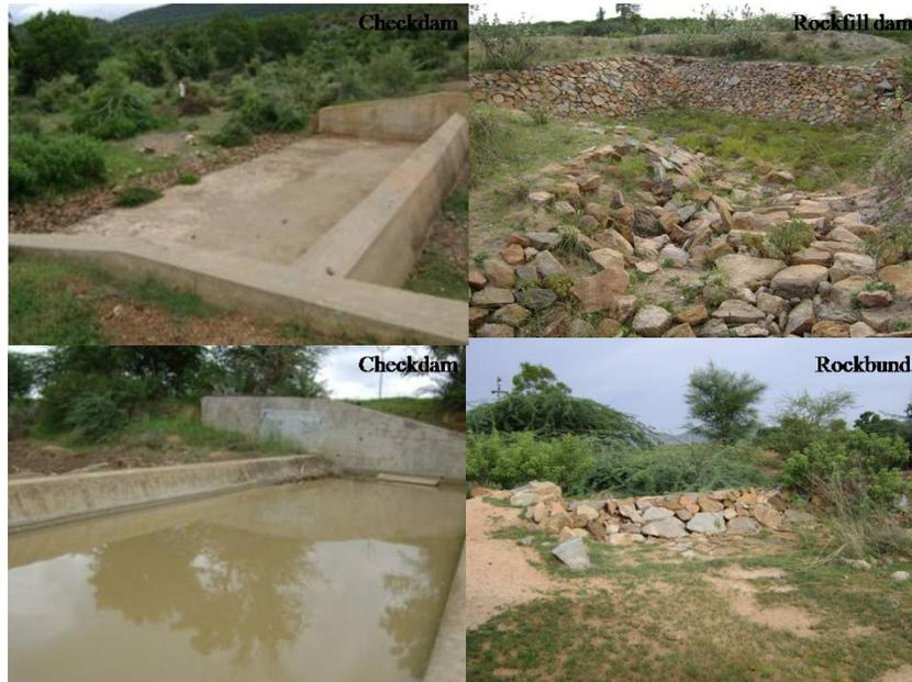
Fig. 1: Different Water Harvesting Structures
