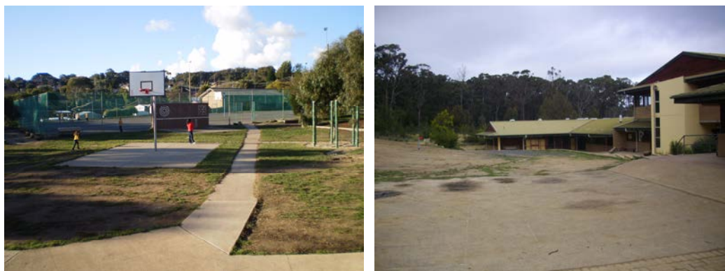
Figures 5 and 6: Example of both primary (Figure 5) and secondary (Figure 6) school playground areas without sun protection from trees
