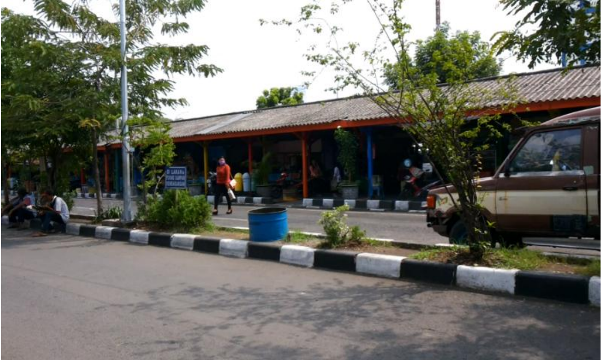
Figure 12. Public transport station at Terminal Joyoboyo Surabaya, Indonesia.
